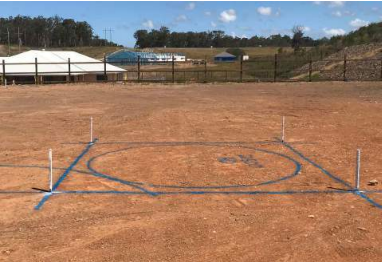
Rainwater System Ground Mark out
