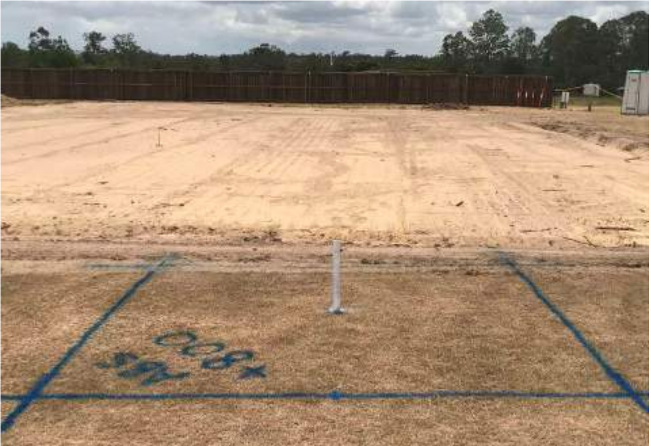
Secondary Wastewater Treatment System Ground Mark out
